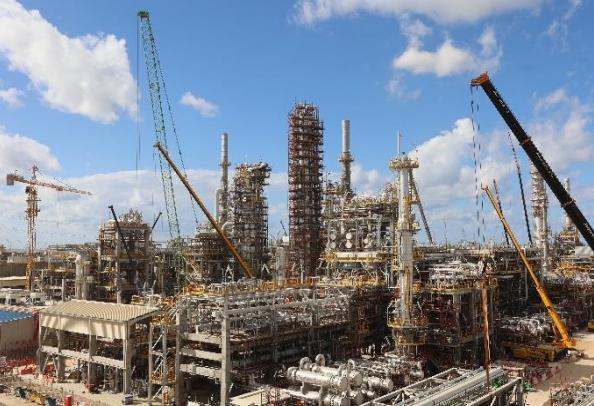
The expansion and modernization Project is a strategic initiative designed to enhance refinery capacity, upgrade existing units, and maximize the production of middle distillates. The project involved the addition of 60,000 barrels per day (bpd) of crude oil capacity through the installation of 5 new process units and the revamp of 10 existing units, producing a product slate that includes LPG, EN228 gasoline, Jet A-1 aviation fuel, EN590 diesel, and petroleum grade coke.
